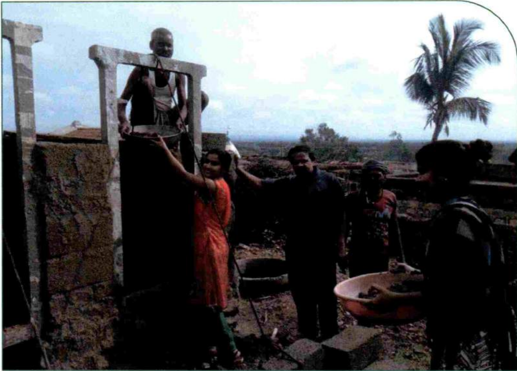
EVENT: Toilets construction under swachhabharatabhiyana at adopted village, Karadigudda (2017-20)
